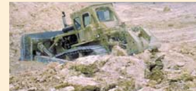
Clearing overburden at Al Jalamid
