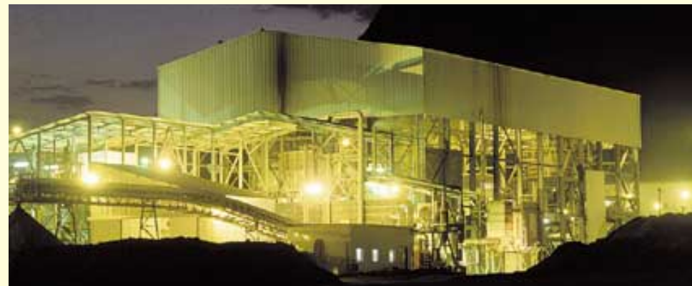
Processing plant at the mine
