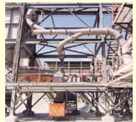
Part of the gold treatment facility
